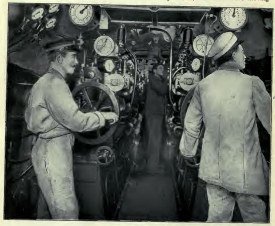
Aboard a submarine - Internal combustion engines.
